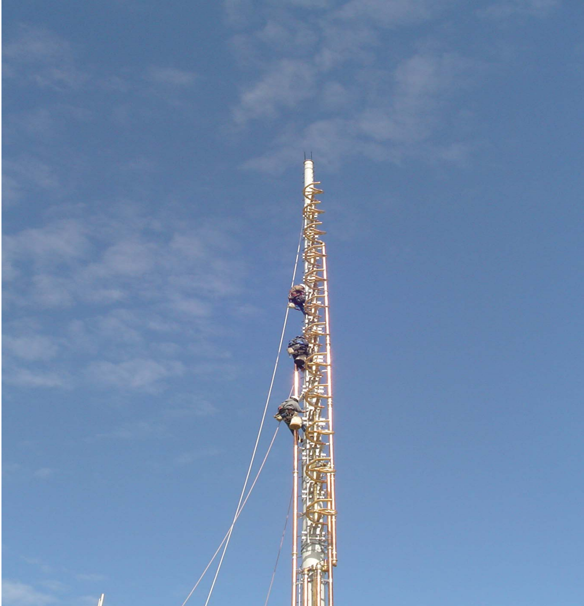
Photo 2: Final assembly of antenna ~ deicer wiring.
